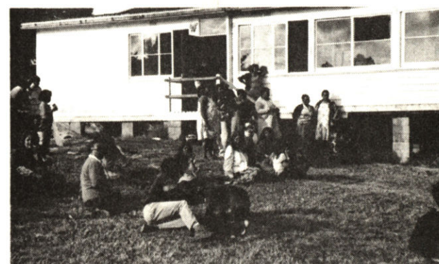
The residents of the Aboriginal settlement of Wreck Bay greeted us outside their school. Note how much it looks like an Indian Affairs school.
