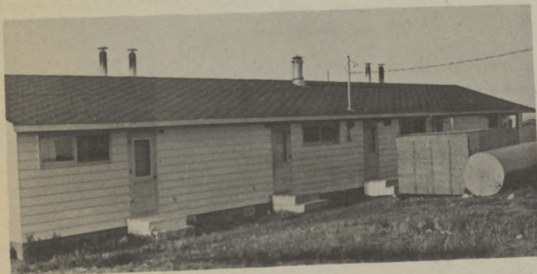
This is a four unit old folks home at Fond Du Lac, Saskatchewan, the first one in the area, built about five years ago by the Fond Du Lac Band. Three homes were released in order to have this old folks home built that particular year. The pensioners, living in the home, pay $40.00 per month for fuel which goes to the Band.
