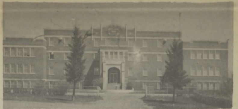
FRONT VIEW: This is how the school looked a few years after its final construction. Its outward appearance has not been changed but there have been a good deal of renovations inside since then.
