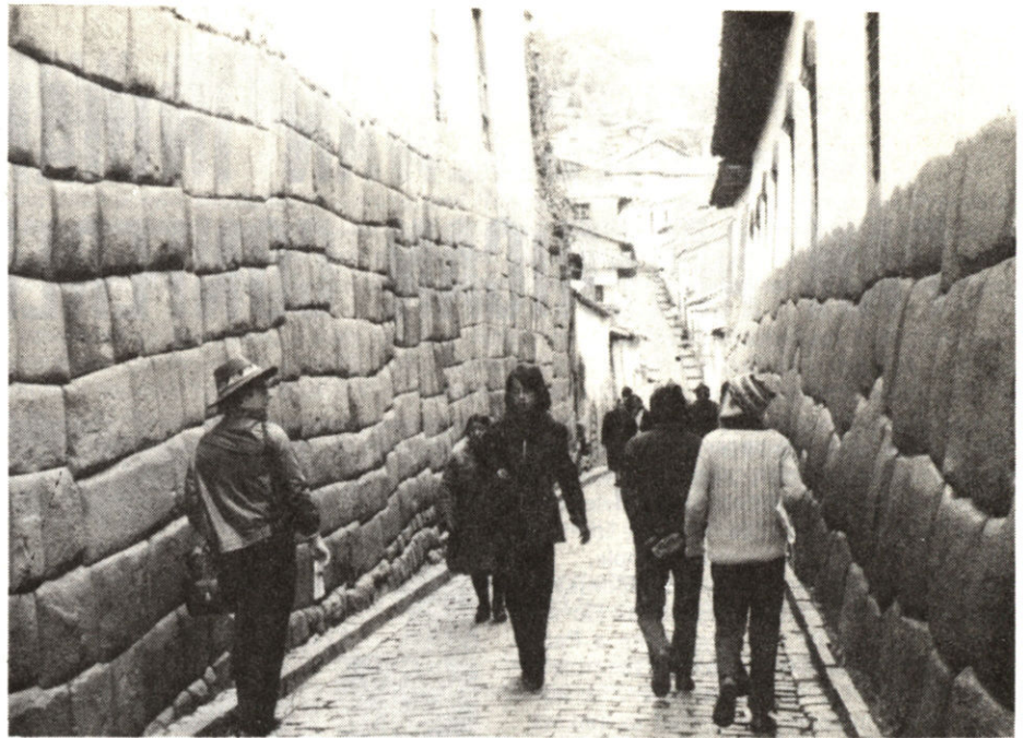
An old Inca Street with the modern city Built around. Cusco has been hit by several major earthquakes. Each time the modern building crumble, but the Inca stone work remains intact.
