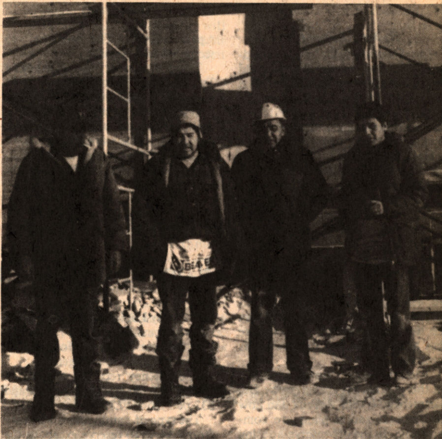
Carpenters at John Smith Reserve building the Community Centre. Left-right, Lloyd Bear, Austin Bear, Lionel Bear, Hubert Bear.
