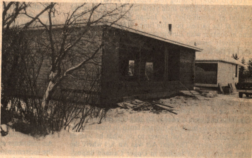
Recreation Hall under construction.
