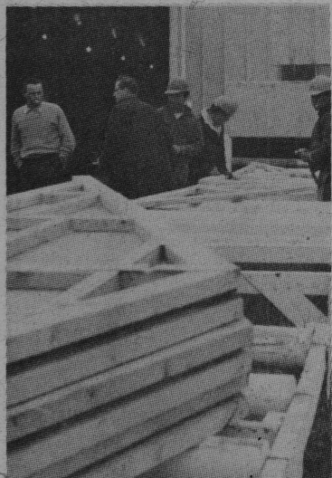
WORKMEN PRE-BUILD A HOUSE SECTION
