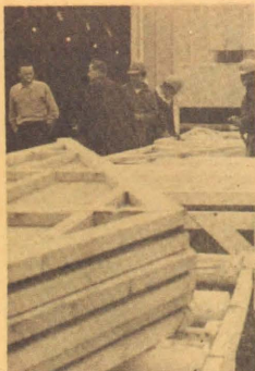
WORKMEN PRE-BUILD A HOUSE SECTION
