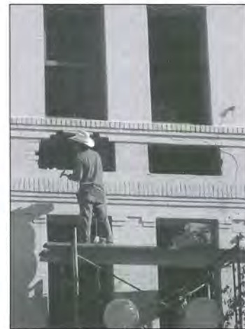
Mason works to repair damage to the Navarro facade.
