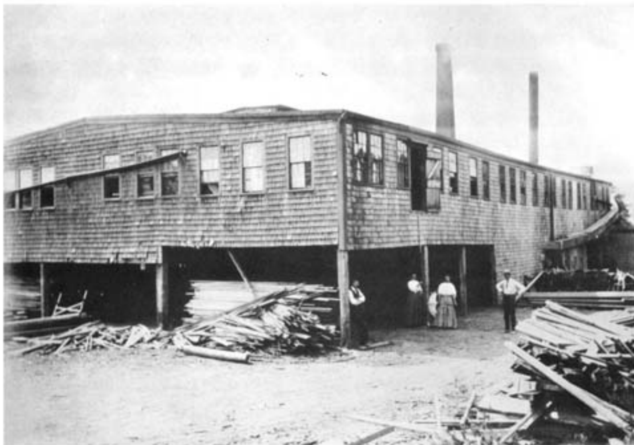
John Foster Lumber Co. Established 1879 (Main St.)
