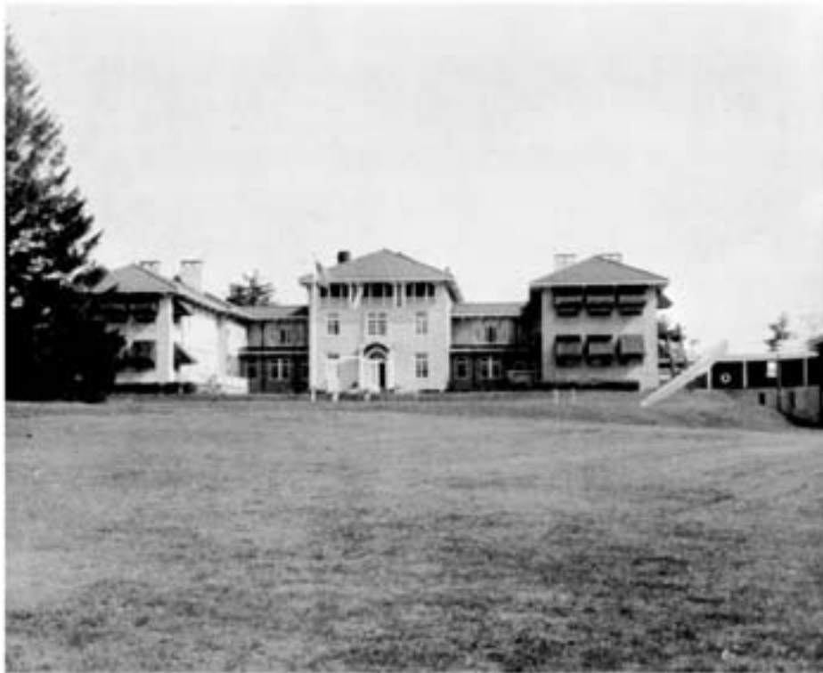
Plymouth County Hospital dedicated May 31, 1919 (High St.)
