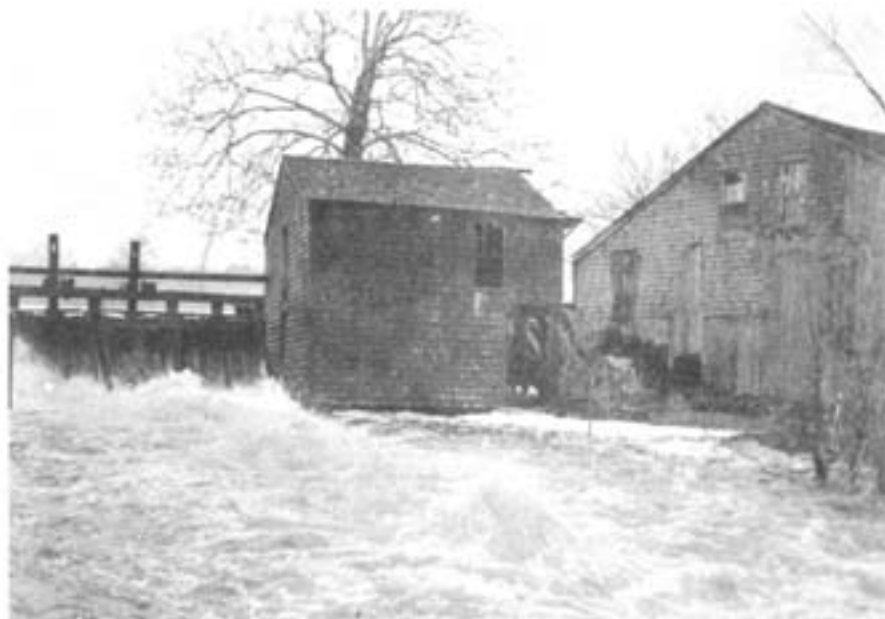
Moore's Saw Mill In Flood Season, site of an original grist mill (1887)
