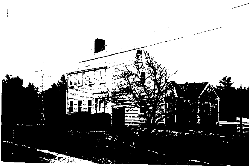
TISDALE WINSLOW HOUSE 94 QUAKER LANE
