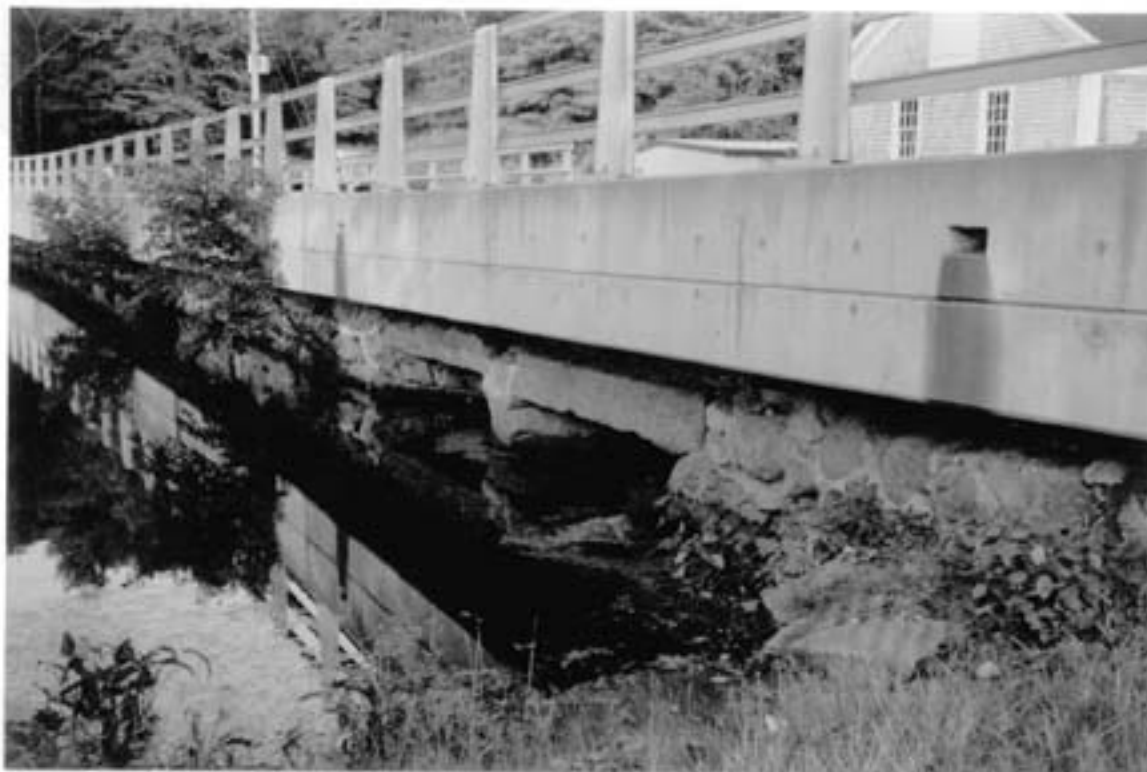
PHOTOS MARY'S POND RD. BRIDGE
