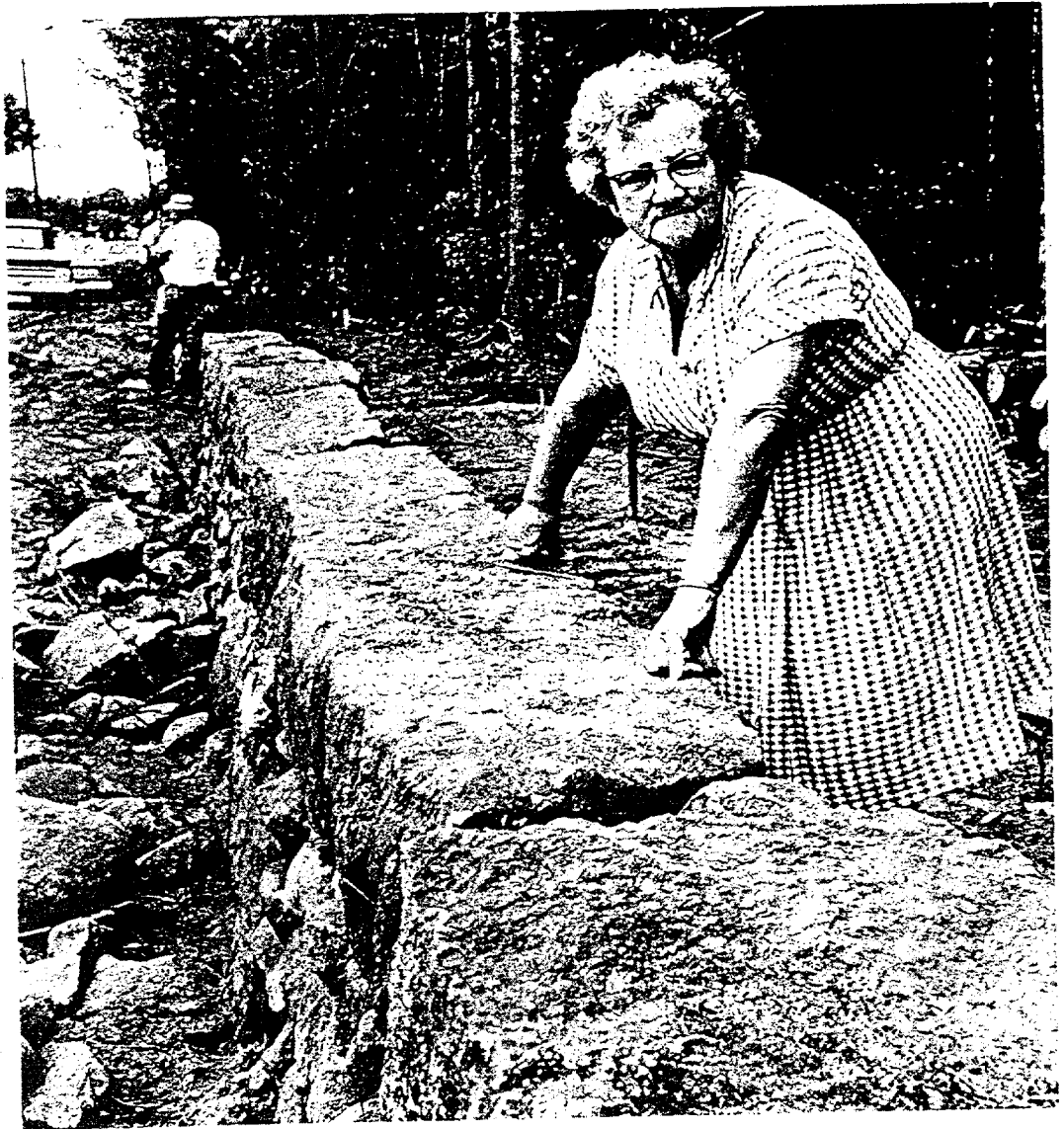
While workmen take a break for lunch, Mrs. Olive B. Winslow checks progress of a double-faced wall being rebuilt on her property on New Bedford Road, Rochester. Field stone and cut granite capping were also used in the original wall built by her ancestor, Zebulon Thompson, when he cleared the land for his homestead, in the early 1800s.
