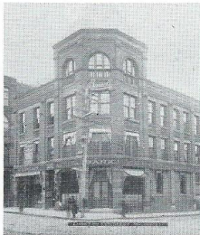
Northeast Corner Main and Centre Streets
