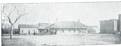
OLD RAILROAD STATION
