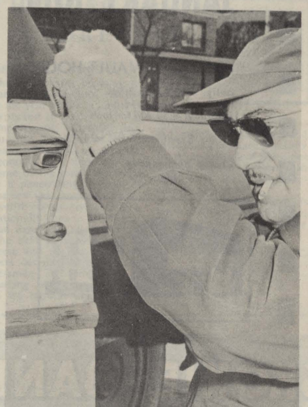
With door ajar, Berger removes the lock so as to obtain the cylinder number. A code book in his workshop will guide him in fashioning a new key even though he has no model to work from.
