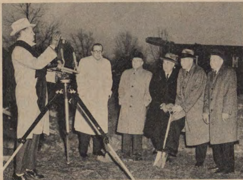
Taking part in the official breaking of ground for an office and warehouse facility at Touby and Tripp Ave. for the AnSCO Division of the General Aniline & Film Corp. are (left to right): B. C. Nicholson, sales supervisor of AnSCO's Chicago district; Harvey Teitelbaum, Fred Teitelbaum Construction Co., Tom Friedman of Friedman, Alschuler & Sincere, architects and engineers; Henry A. Proesel, mayor of Lincolnwood; Harold R. Dean, manager of AnSCO's midwest division; and Marshall Bennett of Bennett & Kahnweiler, industrial realtors.
