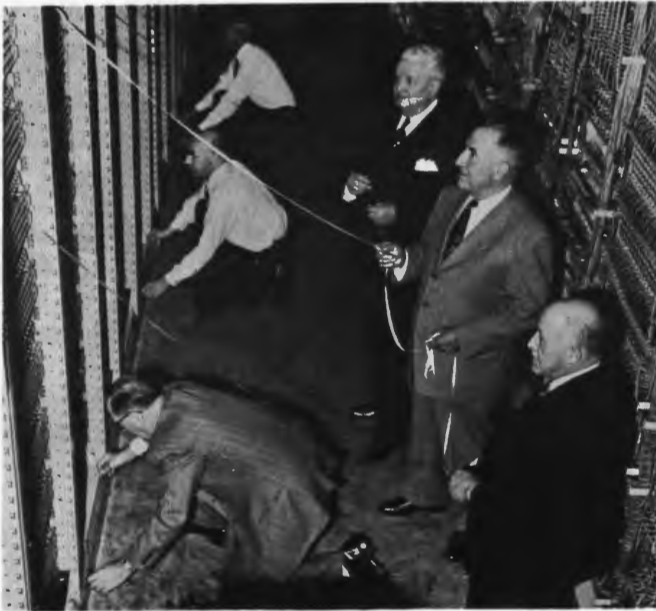
Dial telephone switching equipment was placed in service here October 25, 1952. Standing behind telephone company technicians, ready to pull the ribbons which will place the new equipment in service, are (l to r) Mayors George Wilson of Skokie, Henry Proesel of Lincolnwood and Max Finke of Morton Grove.
