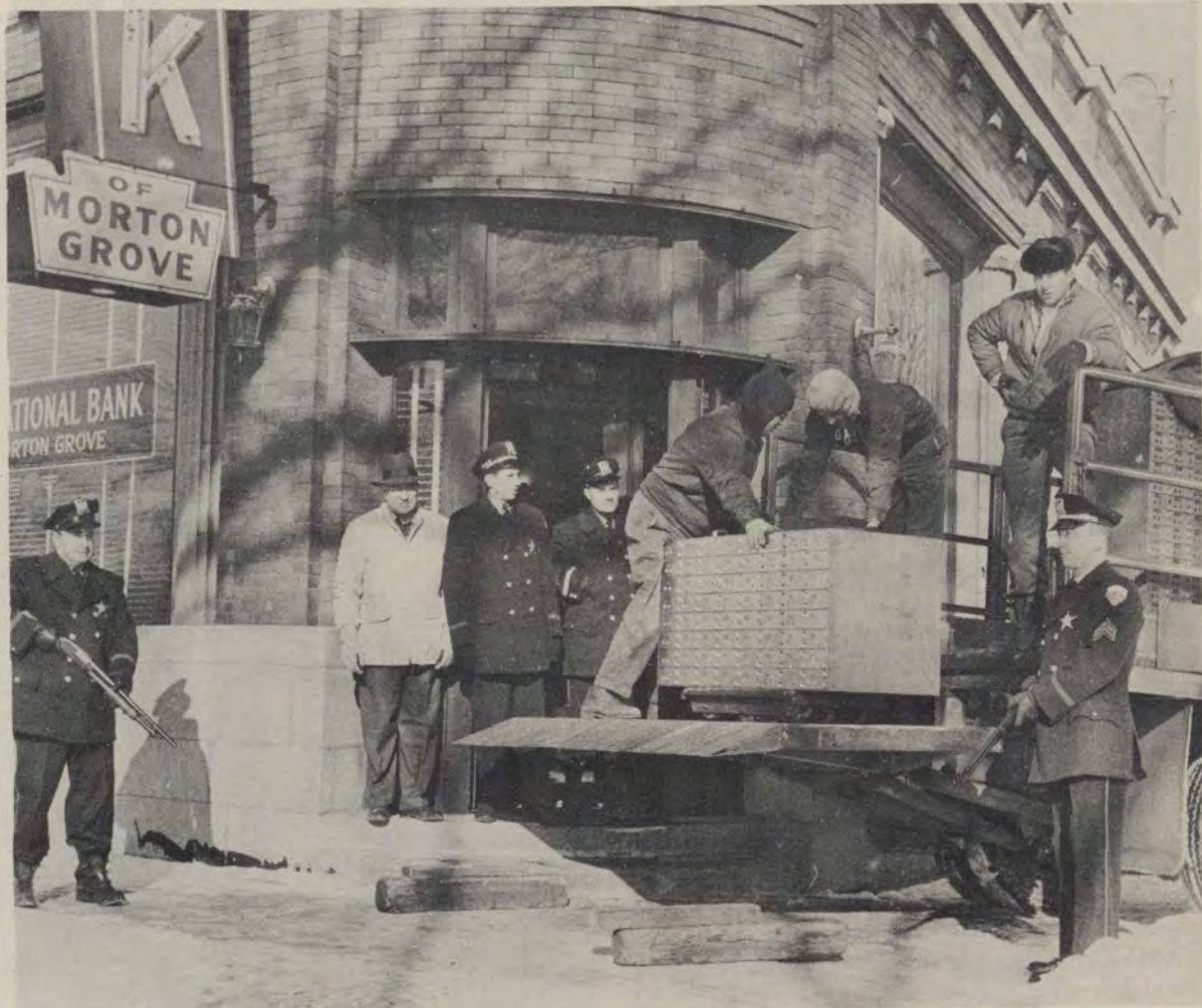
Four Morton Grove police officers stand guard as workmen begin moving safe deposit boxes from the old First National Bank building as it moved this week to new quarters. From left, they are Officer Nick Sirrell, Bank President Roland Dilg, police Chief Mickey Scanlon, Officer Larry Schey. Three workmen load the truck.
