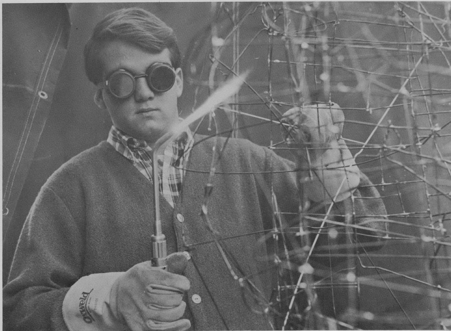
M. Abrahamson welds wire mesh with latest apparatus.
