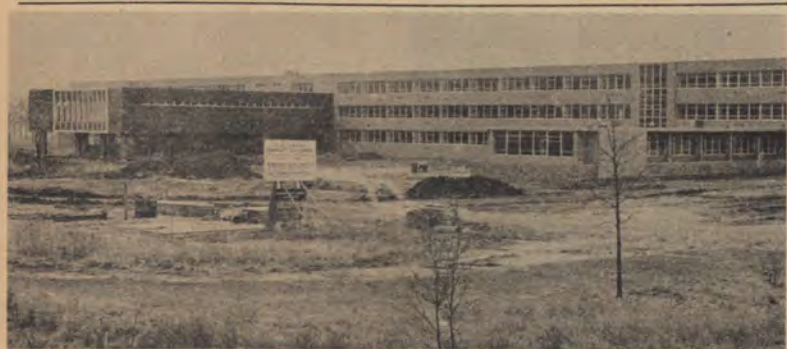
This is a view of the new Niles High West building, awaiting occupancy next fall by freshmen and sophomore classes. Junior and senior classes will continue in present school building. Tax levy increase voted by school district residents Saturday will assure proper facilities and instruction, say school officials.
