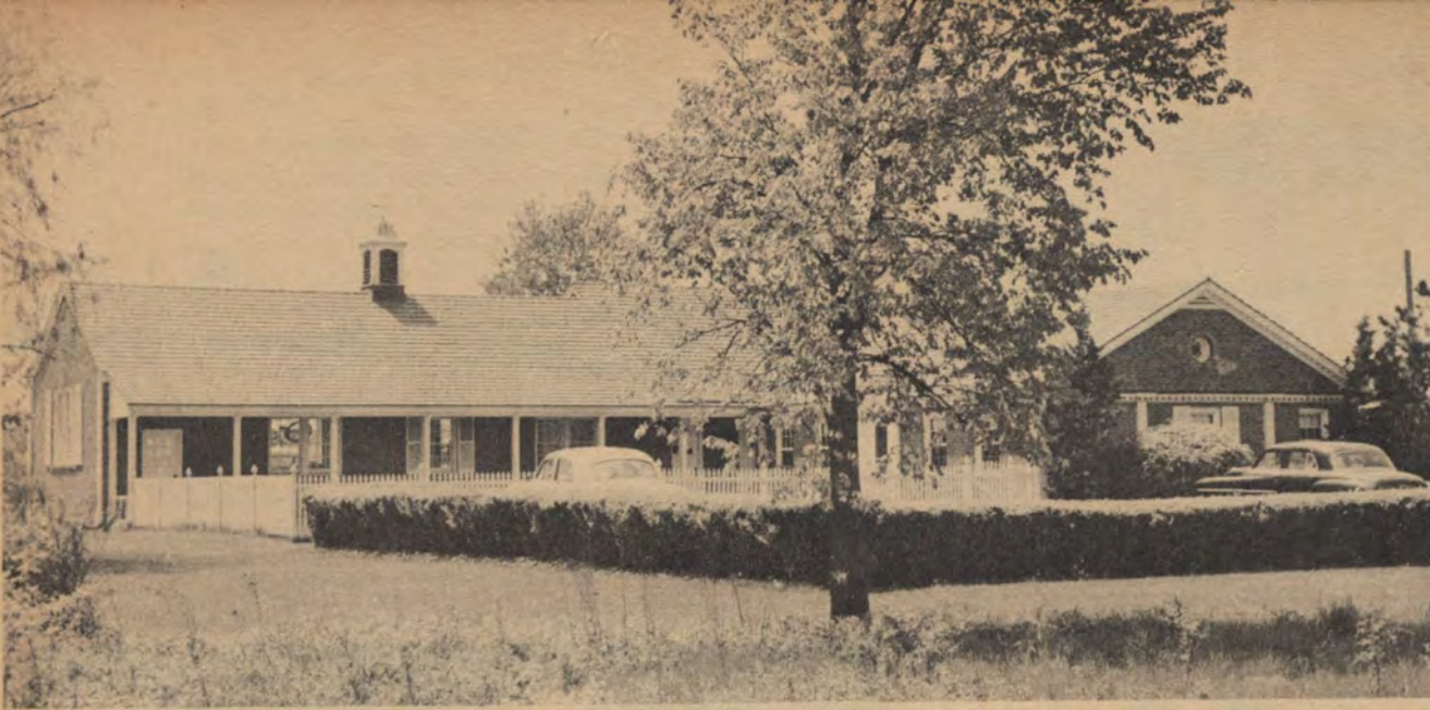
The headquarters of the North Shore Mosquito Abatement District in Northfield.
