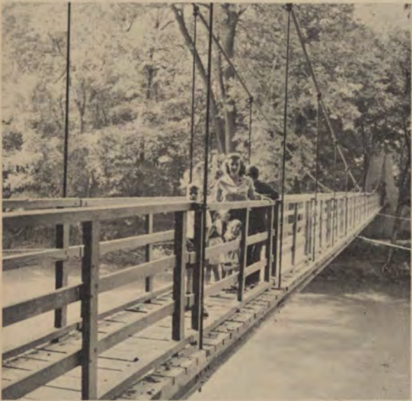
A thrilling stroll is this one - - over Sugar Creek's suspension bridge.
