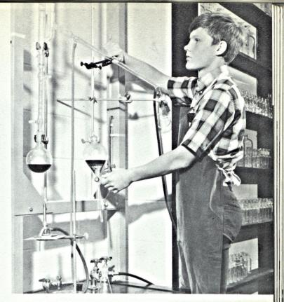
Demonstrating the purification of an organic substance, Richard Rosenquist starts the distillation apparatus.
