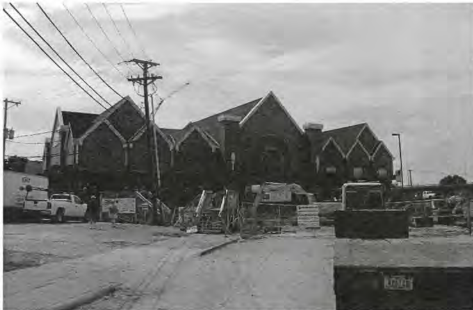
The National Czech & Slovak Museum & Library, NCSML, is pictured July 14, 2011. It has moved 480 feet, pivoted 90 degrees, and is in the process of being elevated 12 feet on to the new foundation/parking garage.
