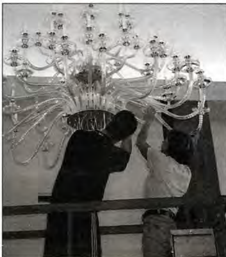
Installation of the new chandelier.
