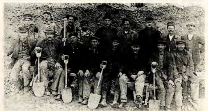
This team of Czech immigrant laborers helped build the river walls for May's Island around 1912. Because cheap labor was needed for public projects, the city was often the first employer of many immigrants.
