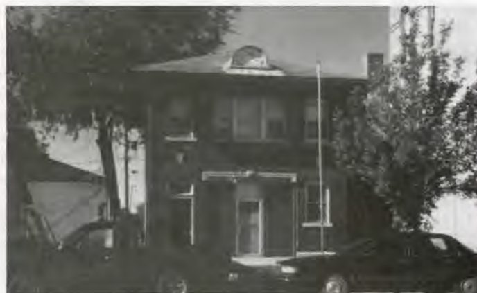
The former firehouse.
