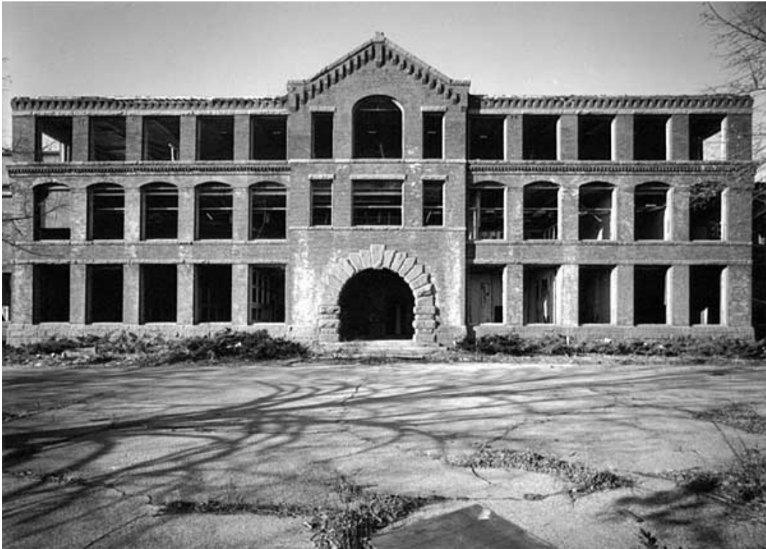
The shell of the Goreham Office Building in 1997.
