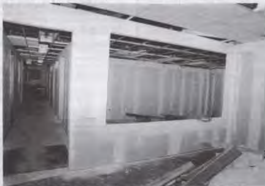
REMODELING UNDERWAY AT NAP'S NEW OFFICES
