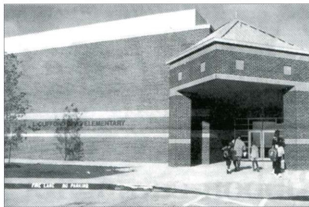
The new L. Clifford Davis Elementary School in Fort Worth, Texas
