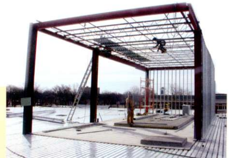
Workers walk the beams on the frame of a utility room atop the ongoing construction of the Kendall Science and Health Mission Center. (photos and story on back cover)
