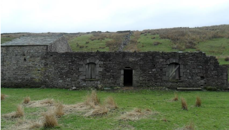
Ruins of Keldside Smelt Mill
