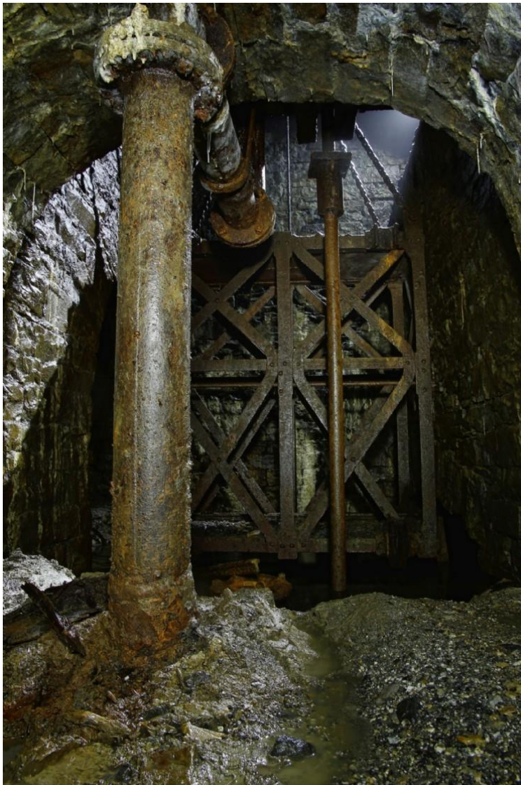
Water Pipe and Shaft Cage; Sir Francis Mine
