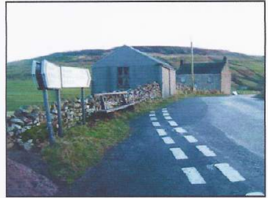
58. Shed, public seat and house on the main valley road
