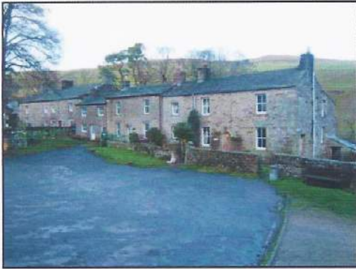
49. North row of the village from the east side
