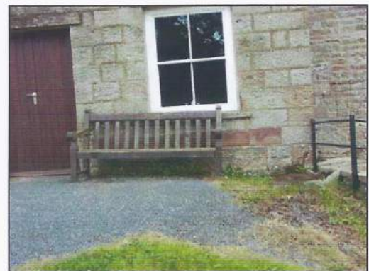
22. Public Hall foundation stones
