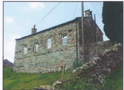
4. Chapel School viewed from north east
