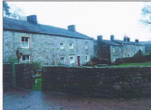
48. North row of the village from the east side
