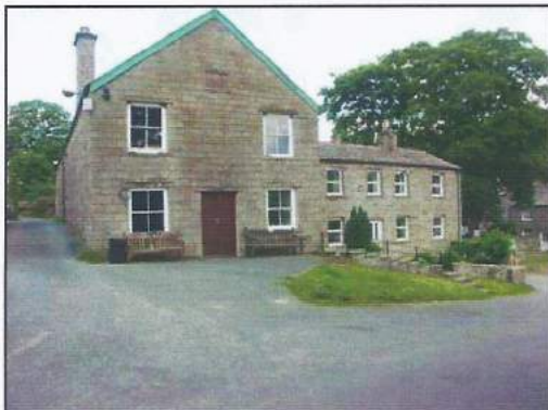
21. Public Hall east end
