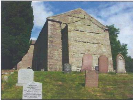
3. United Reform Church viewed from the east
