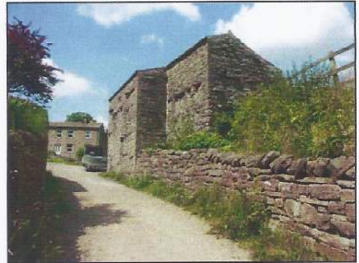
26. Outbuilding looking north west
