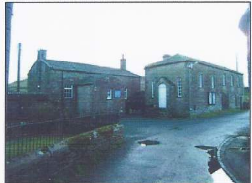
54. United Reform Church and chapel building viewed from the north
