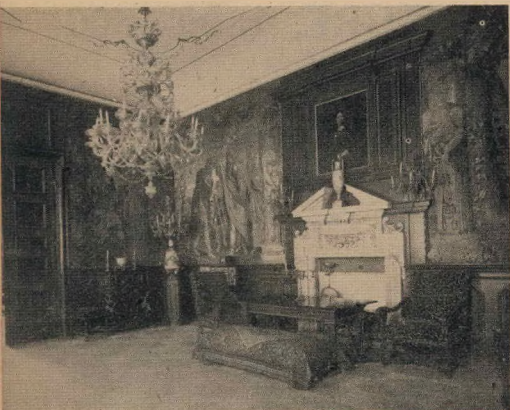
2. A representative chamber, Valdštn Palace, 1623-1630.
