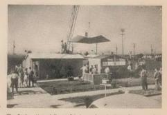
The final section of the roof is lowered on to the walls to complete the house. This model home, which may set a new mode for pustwar housing in the U.S. has a combination living room-dising room, two bedrooms, a kitchen and a bath. Its builder predicts a selling price of \$2,000 when large scale production is started.
