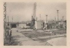
The kitchen and bathroom section is swung into place on the foundation. A plumber is connecting kitchen installations. The front lawn has been dug up and some shrubs planted. Other shrubs (far right) are ready to be transplanted to the grounds by a landscape gardener working with the construction erew.
