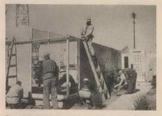
The main wall, with door attached, is fastened to the foundation by workmen. The bedroom (tright) is in place and the furniture has been moved in. Through the window (centre) a man may be seen laying the living room rug. Al right, gardeners continue work on the grounds.
