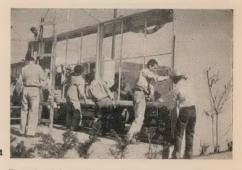
The main window section, complete with blinds and drapes, is lowered into piace. The gardeners have finished landscaping the grounds. (Note shrubs in foreground.) Wallpaper was pasted on the walls when the house was prefabricated. At this stage of assembly, the intrifor was almost complete.
