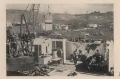
Workmen and the tenants of the new house move in furniture and set the living room in order while a crane lowers a window section, complete with curtains, into place. The plumber (left) has finished connecting the kitchen installations.
