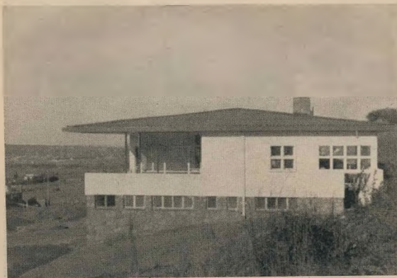
West Elevation, showing low-pitched, asbestos cement roof, painted black, with broad eaves overhang.
