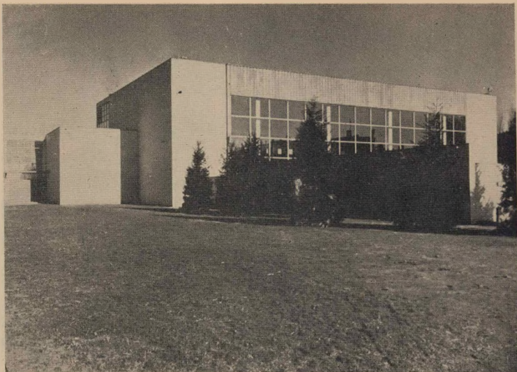
General view of the swimming pool building. Walls of buff brick enclose a steel frame; copper spandril over window. BELOW: The interior.
