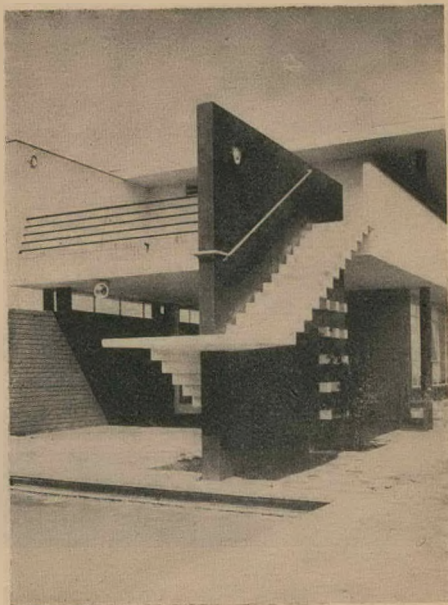
THE CANTILEVERED STAIRS providing an external communication between lounge and bedroom and serving as a diving platform for the swimming pool.
