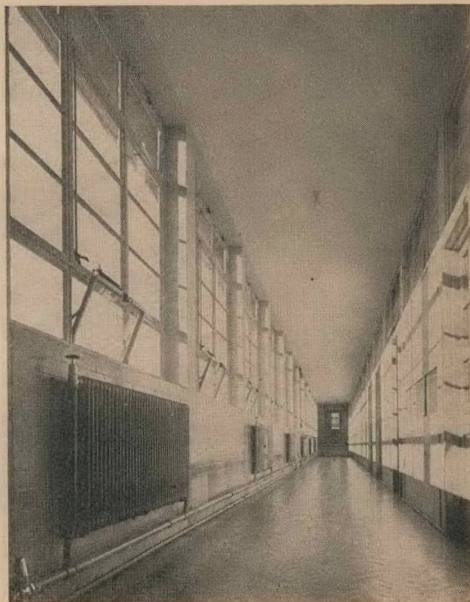
BELOW: View of the first floor corridor in the Science wing.
