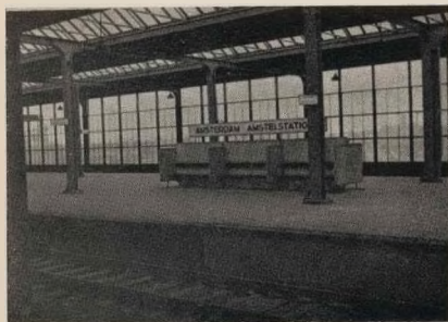
View looking across the platforms.
