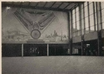
General view of the main concourse.
