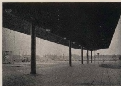
The covered taxi stand at exit.
