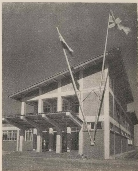
The portico to the main entrance hall, Administration Block. The panel walls are in blue-grey face bricks, windows are painted white, external wood work blue, the portico and the underside of eaves orange, reflecting the colours used in the company's catalogues. Roof is corrugated asbestos cement.
