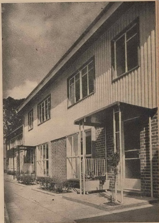
THE TWO EXPERIMENTAL STEEL HOUSES AT NORTHOLT OF THE BRITISH IRON & STEEL FEDERATION
