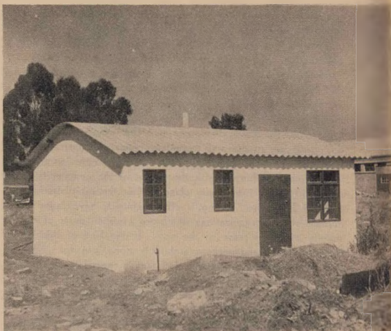
EXTERIOR VIEW. THE HOUSE IS FINISHED WITH ROUGH CAST EXTERNALLY.
