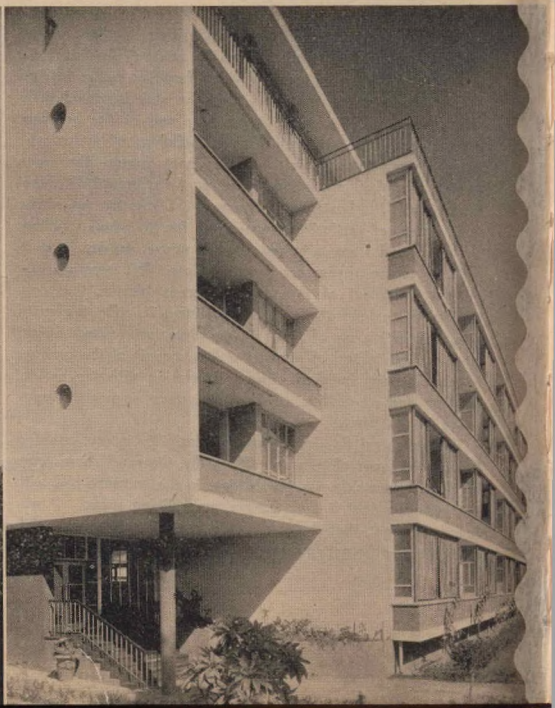
beyond; and RIGHT: A detail of the north facade, where deep recession shades and protects the rooms behind. The combination of white plaster, red bricks, black and red railings and gaily coloured blinds give the building a bright and attractive appearance which, with its broad sweep of well-tended gardens, creates in this scheme an atmosphere as attractive as it is unexpected so near the centre of the city.
