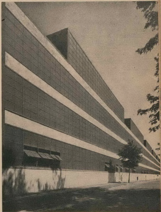
DIESEL ENGINE PLANT.
