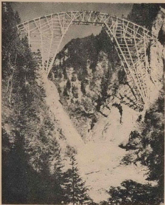
BRIDGE OVER SALGINA-TOBEL. SWITZERLAND, by MAILLART.
