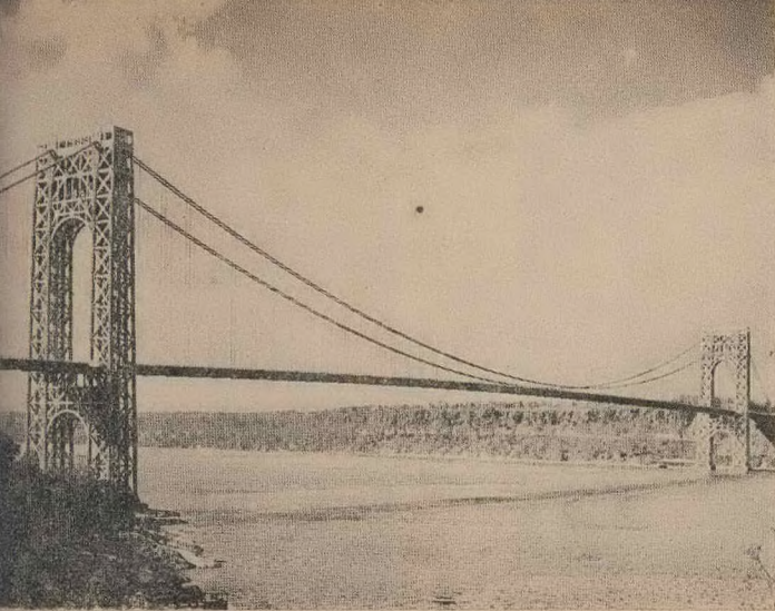
GEORGE WASHINGTON BRIDGE, N.Y.C. Engineering beauty. The pylons were to have been sheathed in masonry, which was subsequently omitted when the beauty of the structural steel frame was apparent.
