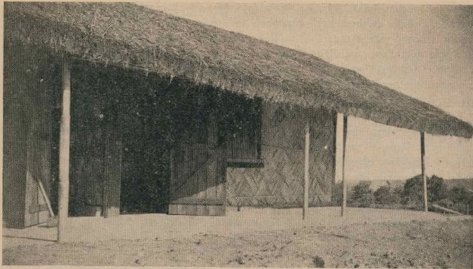
1. BAMBOO BUNGALOW. General view of the front, showing the deeply over- hanging roof of the ver- andah.
