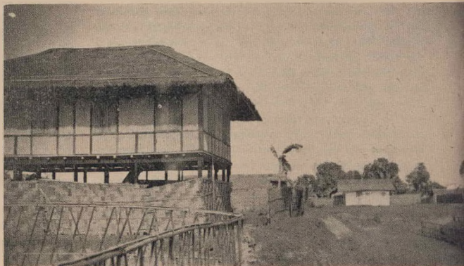
5. A raised timber framed bungalow with Cami plastered walls. This building also illustrates the use of nets of cross-woven bamboo slivers at ridge, hips and eaves to secure the thatch of the roof.
