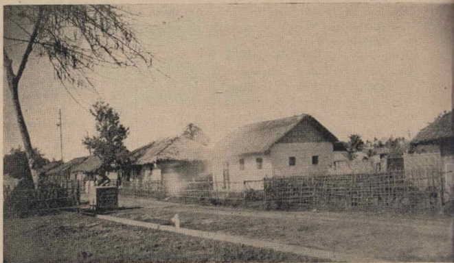
4. BAMBOO HUTS, showing Jeng leaf roofing on the third hut, and a suggestion of the hogsback roof, common in East Bengal, on the hut immediately behind the figure in the middle distance.
