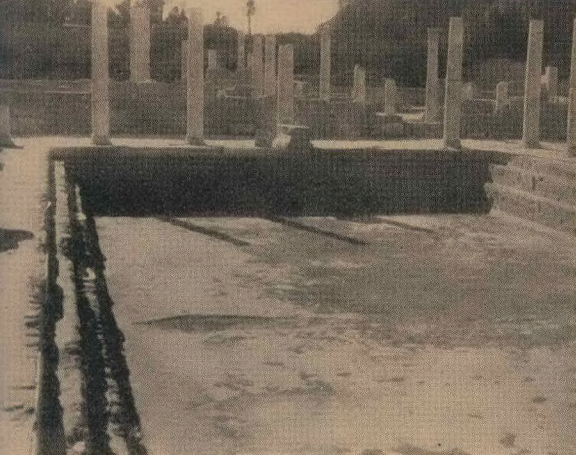
9. GENERAL VIEW OVER FRIGIDARIUM, LOOKING WEST.
