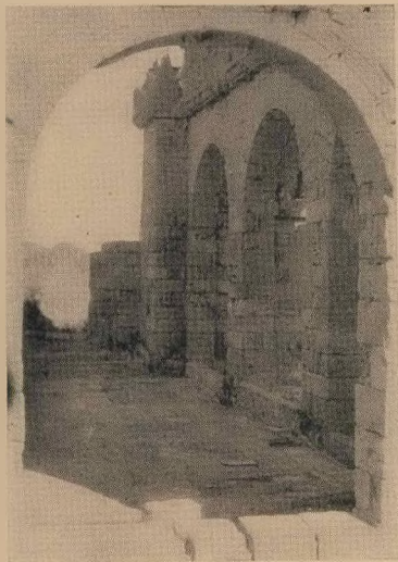
11. VIEW OF THE SOUTH WALL OF CALIDARIUM.
