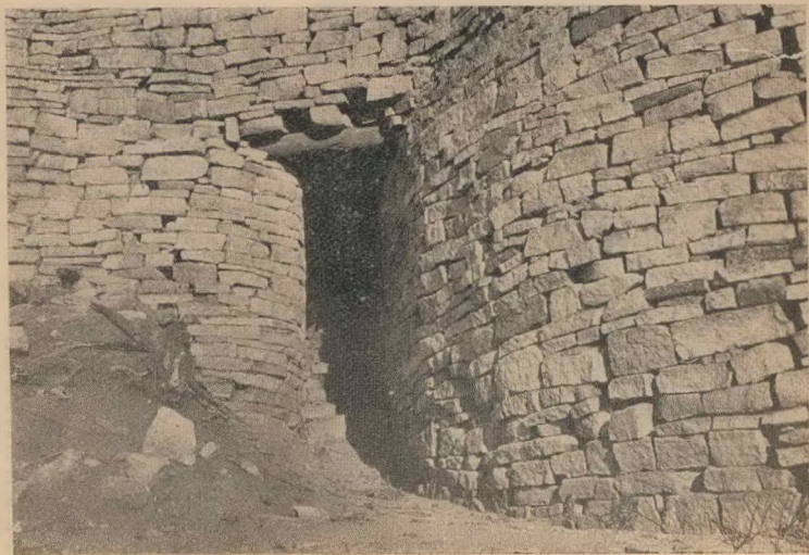
Fig. 8. Covered entrance, showing lintel and lack of bonding, Acropolis, Zimbabwe.
