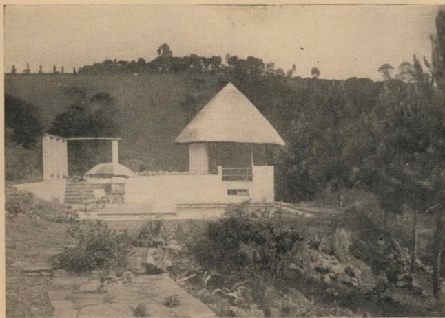
THE SWIMMING POOL AND GARDEN SHELTER: The L-shaped pool measures 40 feet by 15 feet, finished with a dark brown brick-on-edge surround. The pool is painted light blue. The shelter and change rooms below are built of 9-inch brick walls, plastered and whitewashed.
