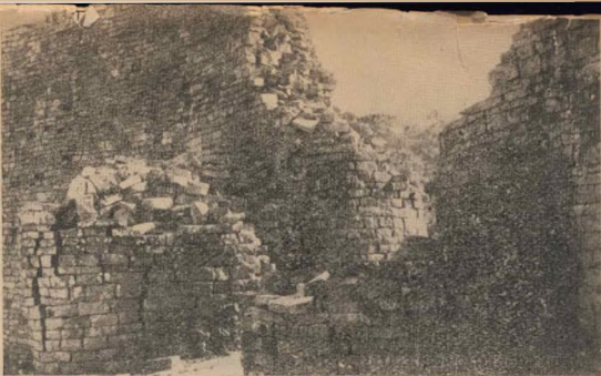
Fig. 6. View showing lack of bonding and imminent collapse of wall, the West Entrance of the "Elliptical Temple," Zimbabwe.
