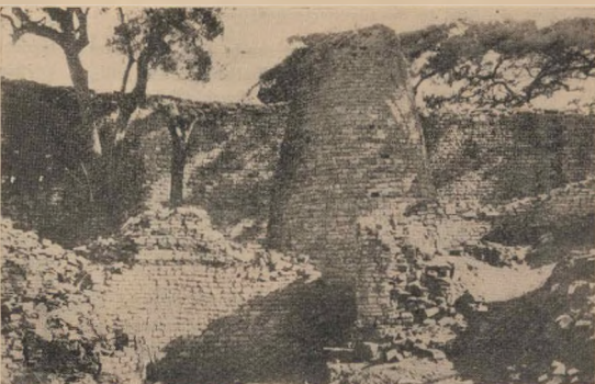
Fig. 7. Conical Tower, banded decoration in wall in left foreground, and general lack of bonding, Zimbabwe.
