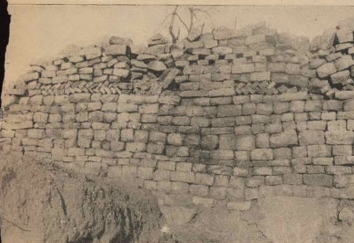
Fig. 11. Khami Ruins, Rhodesia, showing herring-bone and check pattern. Note defective bonding.
