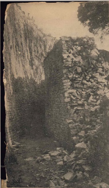
Fig. 5. View of collapsed wall at Zimbabwe, showing external "skin" and in-filling.
