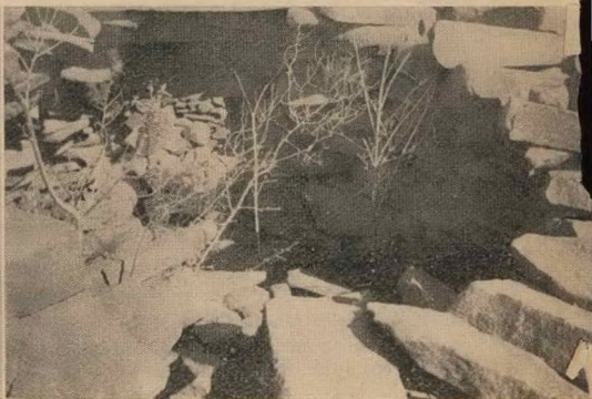
Fig. 16. Collapsed hut, showing corbelling, Steynsrust, O.F.S.
