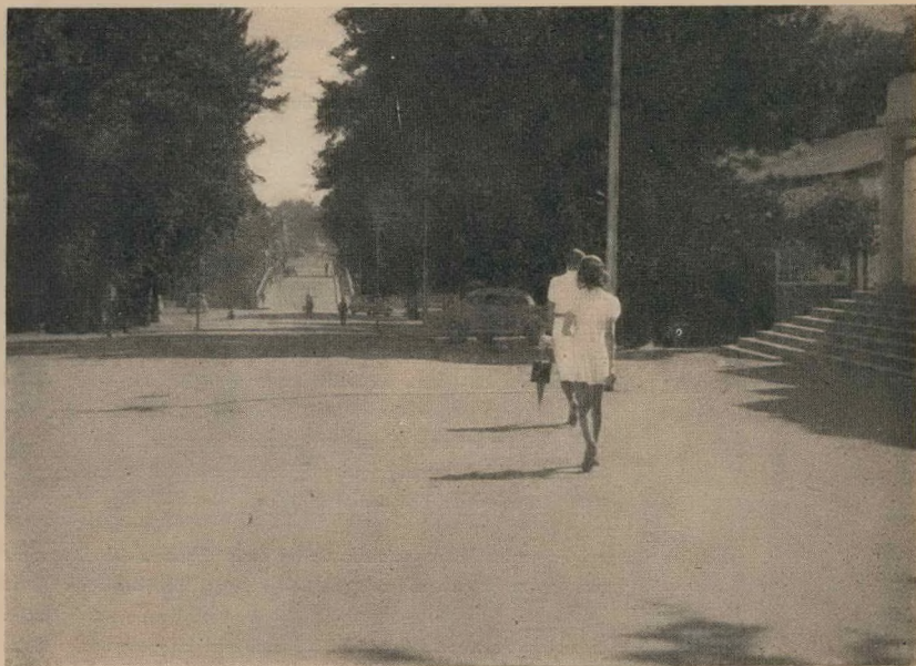
Voortrekker Street, Ceres. A view looking east over the bridge of the Dwars River from the Town Hall.
