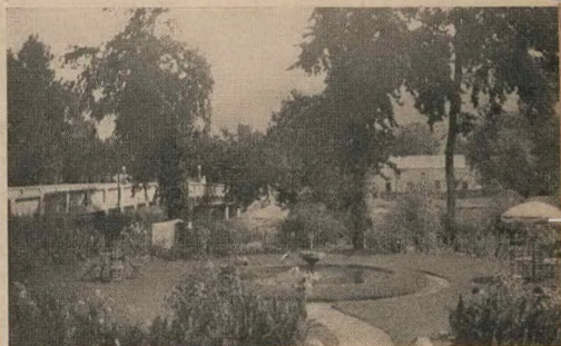
The Dwars River Bridge seen from the Tea Gardens.
