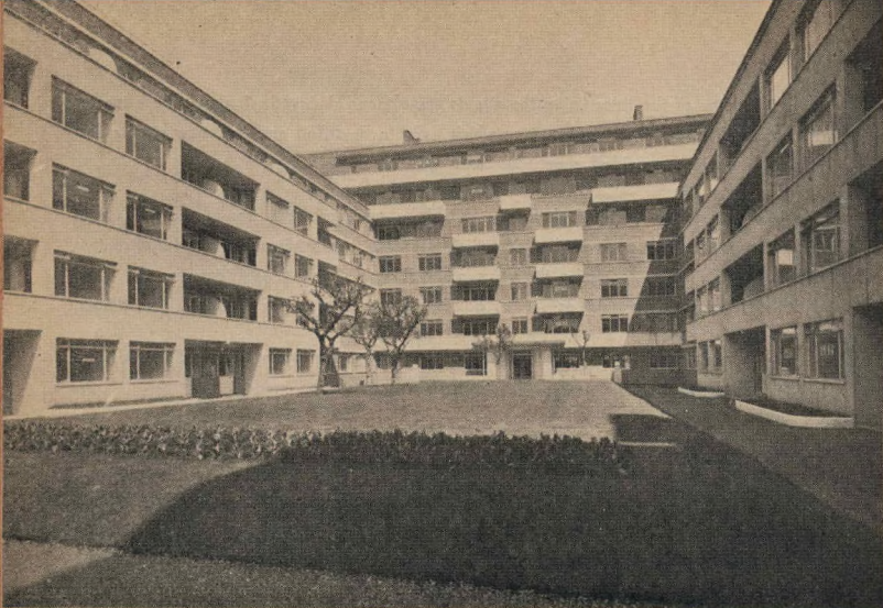
FLATS IN PUTNEY, LONDON, by Frank Scarlett, Architect. The wide windows between balconies, looking out over the grassed court, give a feeling of space, and are combined with an attractive simplicity of line and composition.
