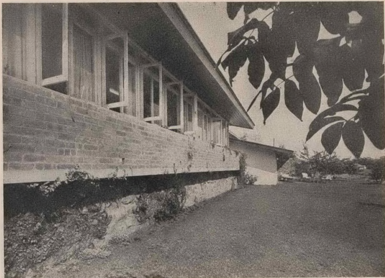
View of the North front of the Bedroom Wing, showing the raised floor level arranged for privacy of the bedroom wing.
