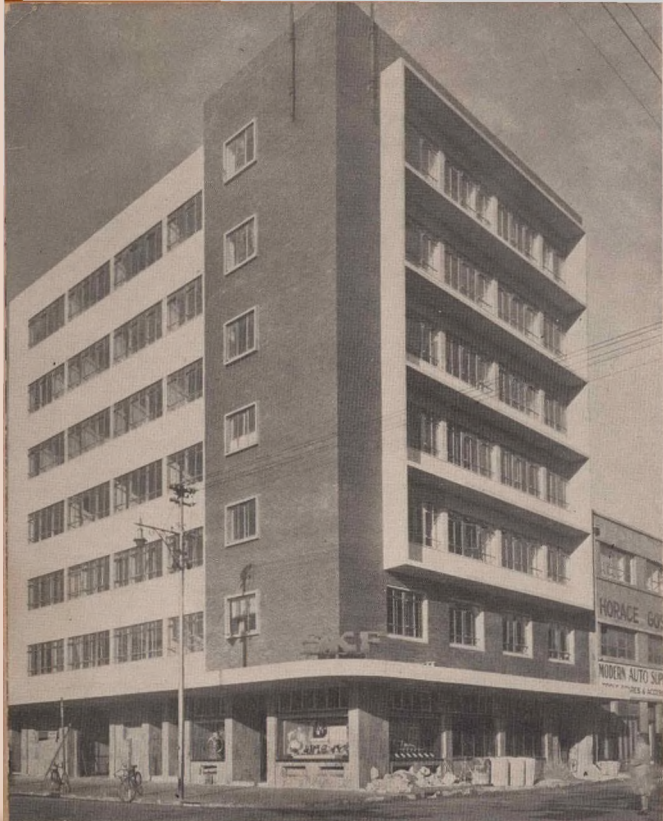
6. S. K. F. BALL BEARING COMPANY BUILDING: 1950, by Chris Niell, Architect. This is one of the better well-finished recent additions to Johannesburg's office buildings. The two principal forms in the superstructure are treated with terrazzo facing slabs and face brickwork. This strong differentiation is typical of a good deal of post-war work, and in this case virtually separates the building into two component parts which thereafter remain unreconciled. The building thus does not achieve an overall sense of unity.
