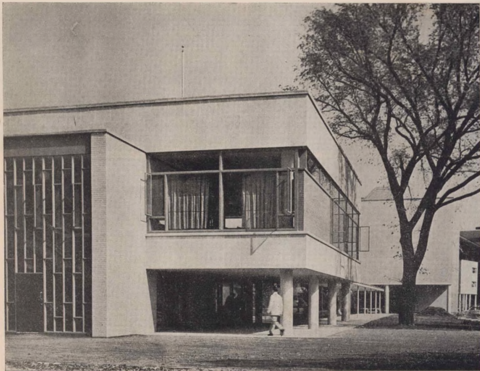
LEFT: The rear wall of the fireplace in the Swaine Room with brick sculpture by Josef Albers. BELOW: Detail of the Harkness Commons, looking East. Limestone facing slabs and light coloured facing bricks are used on the exterior surfaces.
