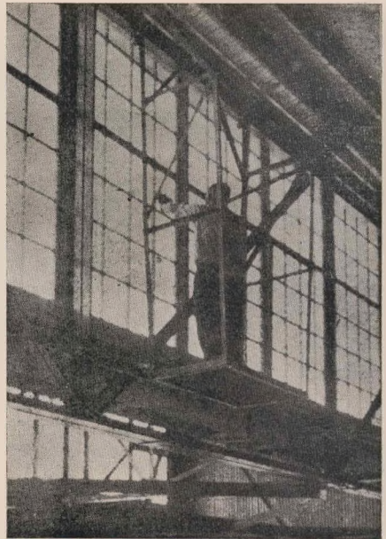
Fig. XIII. The cleaning of sawtooth glass areas is made simple and safe by the use of a mobile cage, which can be moved by the window-cleaner as he works. The cage runs on grooved pulleys along the upper monorail, and guide pulleys in contact with the lower rail keep it steady during the cleaning operation.
