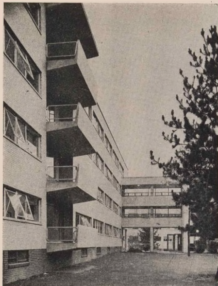
Detail of block 4 looking south. Light coloured facing bricks are used on exterior surfaces, with limestone facing on the connecting link between this building and block 3 seen at right.
