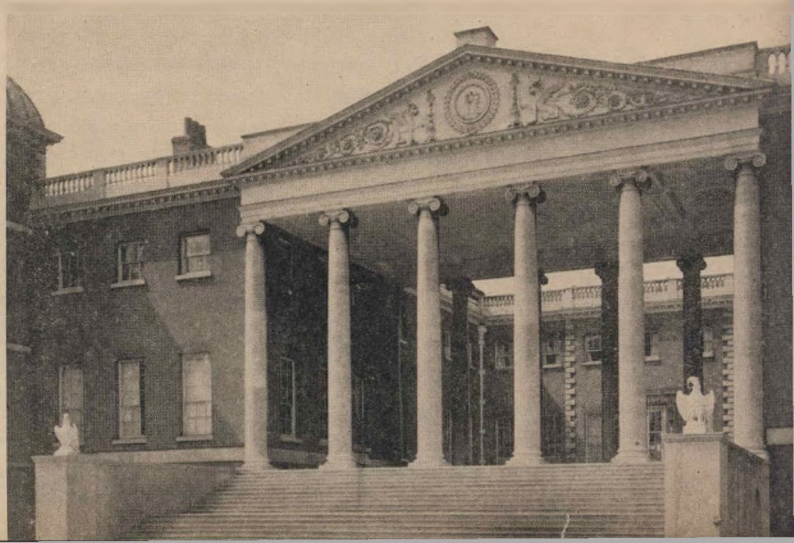
Osterley Park, Middlesex, showing the magnificent double colonnade portico of Portland stone, which reveals the influence of Palladio. Osterley is the seat of the Earl of Jersey, and was rebuilt by Adam in 1761.
