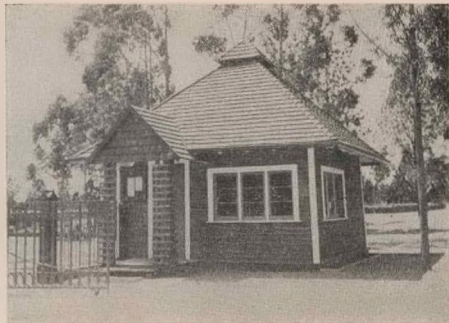
5. Watchman's Lodge just after erection in 1937. Roof of P.patula shingles impregnated in a creosote-fuel oil mixture.
