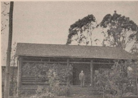
3. North face of cypress roof of log cabin after 18 years' service. Note badly weathered raw of untreated red cedar shingles along centre of roof.
