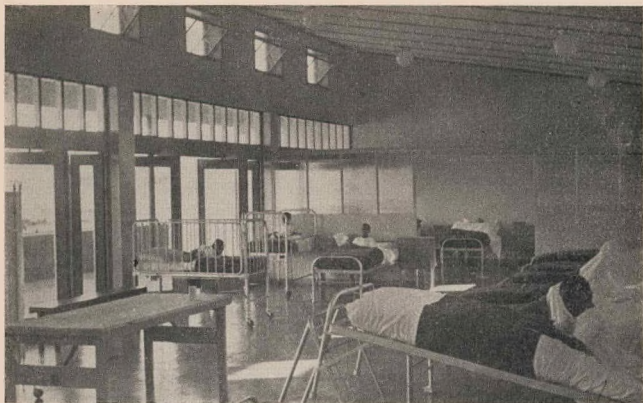
LEFT: View across the Native Dormitory, showing the generous verandah space, extending the length of the dormitory and having an eastern aspect.
